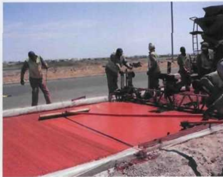
The City of Cape Town decided on a textured broom finish for the BRT network after considering various options.
