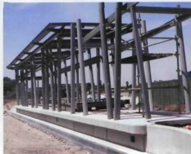
One of the BRT stations under construction.
