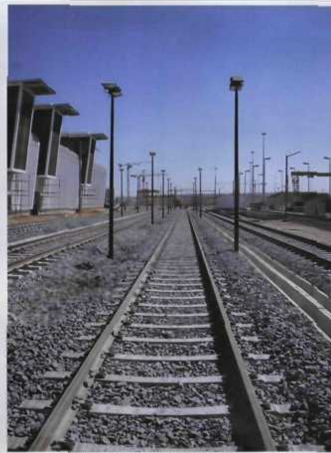
Ballast being compacted during the mainline construction.
