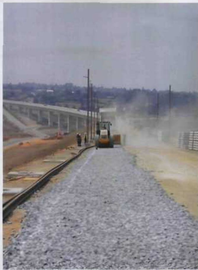
Ballast at the Gautrain Midrand Depot (north end looking south).
