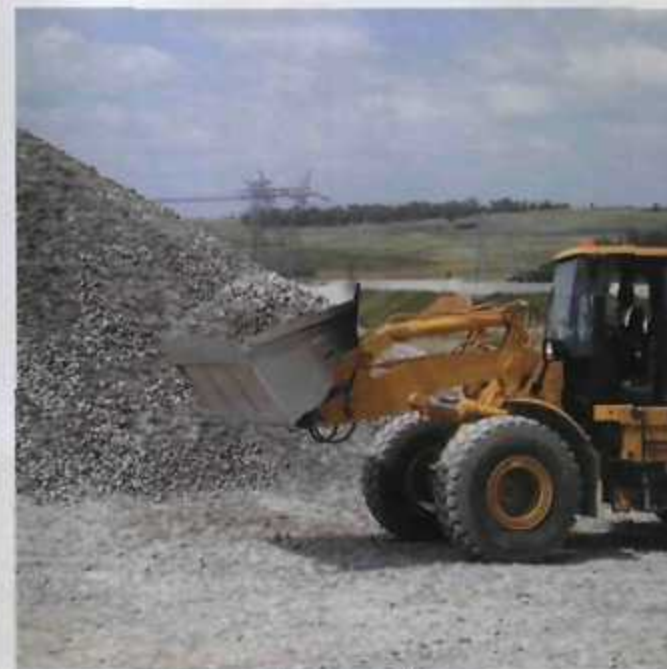
Ballast being loaded.
