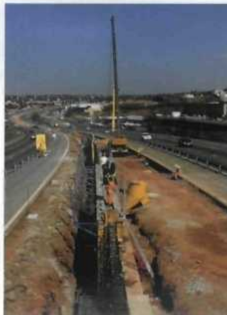
BELOW Workers prepare reinforcing bars and shuttering for a concrete pour
