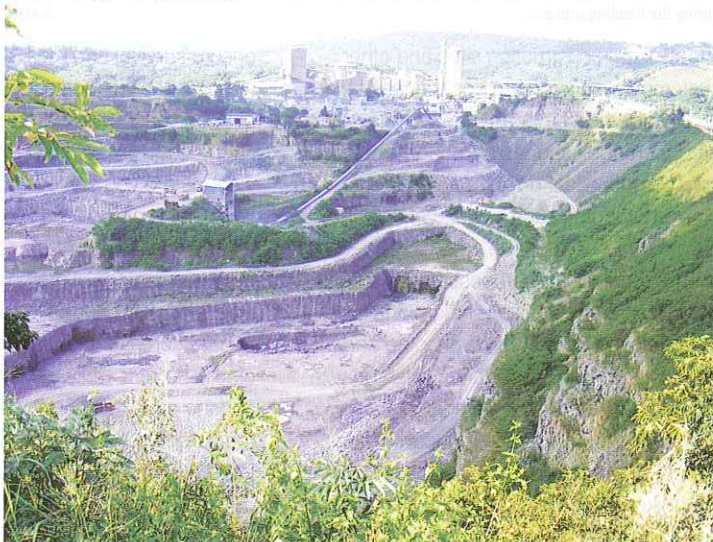
An overall view of Coedmore Quarry.
